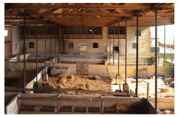
Machine-sawn softwood was commonly employed for roof trusses in the 19th century, combined with wrought-iron bolts and rods and the use of cast iron columns. It is here used in a revolutionary design covered yard of the 1860s. Photo © Mike Williams/ English Heritage
