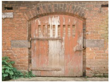
Plank and ledged doors are typical, and are hung off heavy frames or hinged directly into masonry walls. Photo © Mike Williams/ English Heritage
